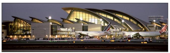
Nine of TBIT's 18 gates can accommodate the new-generation Category VI aircraft such as the Airbus 380 and Boeing 747-8 Intercontinental jets. A-380 aircraft are served by three passenger boarding bridges (one reaching an aircraft door on the upper deck) for efficient boarding and deplaning. Each gate is equipped with a Safegate Advanced - Visual Docking Guidance System.
